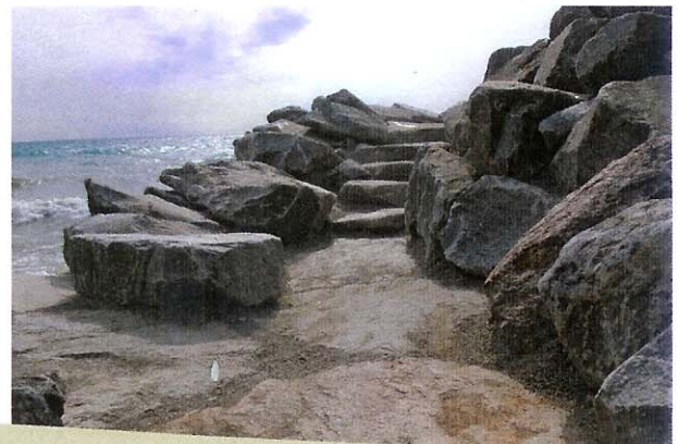
Special placement allows for the addition of stairs and walking paths that provide access along the site (below).
