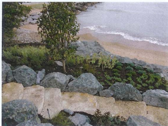
Winnetka bluff restoration project... more to come.
